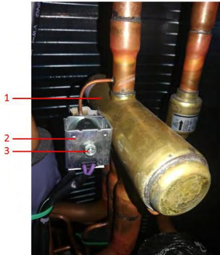
1 --- 4-way valve    2 --- 4-way valve coil    3 --- Screw
