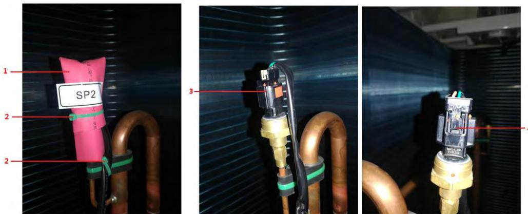
1 --- heat-shrinkable sleeve 2 --- high temperature wire tie
